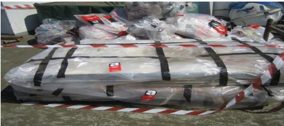
Figure 3. Packaging of asbestos containing material 8
